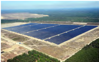
Solar power plant Lieberose, Germany
